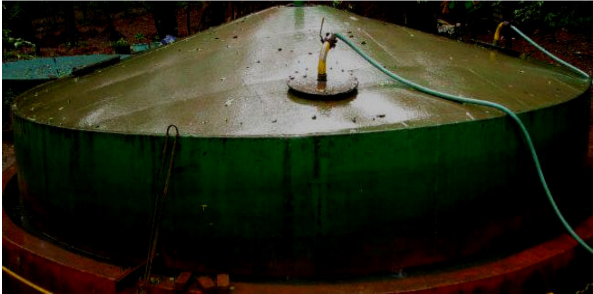
Biogas Plant at college
